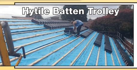
In today's market where block sizes are becoming smaller, the options for loading a roof from all sides are limited. In these situations, the Hytile Batten Trolley can be a big advantage in speed and energy saving. Just load up the trolley and your tiles are transported from one end of the roof to the other with a minimum of physical effort.
