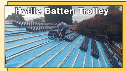
In today's market where block sizes are becoming smaller, the options for loading a roof from all sides are limited. In these situations, the Hytile Batten Trolley can be a big advantage in speed and energy saving. Just load up the trolley and your tiles are transported from one end of the roof to the other with a minimum of physical effort.
